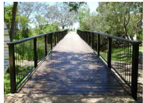
CONDAMINE BRIDGE - PRECEDENT IMAGE
