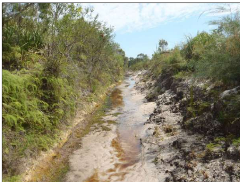
Plate 2.3 Central drain showing lack of macrophyte or sedge cover and steep partly eroded banks
